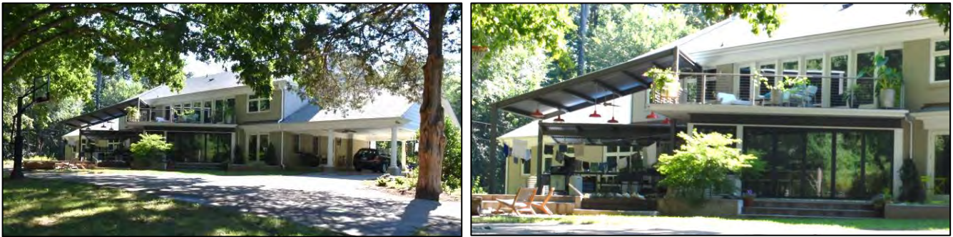
Figure 151: View of rear (western) elevation with original carport in place and modern kitchen addition
