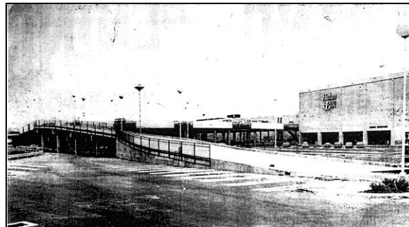
Figure 125: Hudson Belk with ramp to upper parking deck at left and southwest elevation at right (News and Observer, August 2, 1972)
