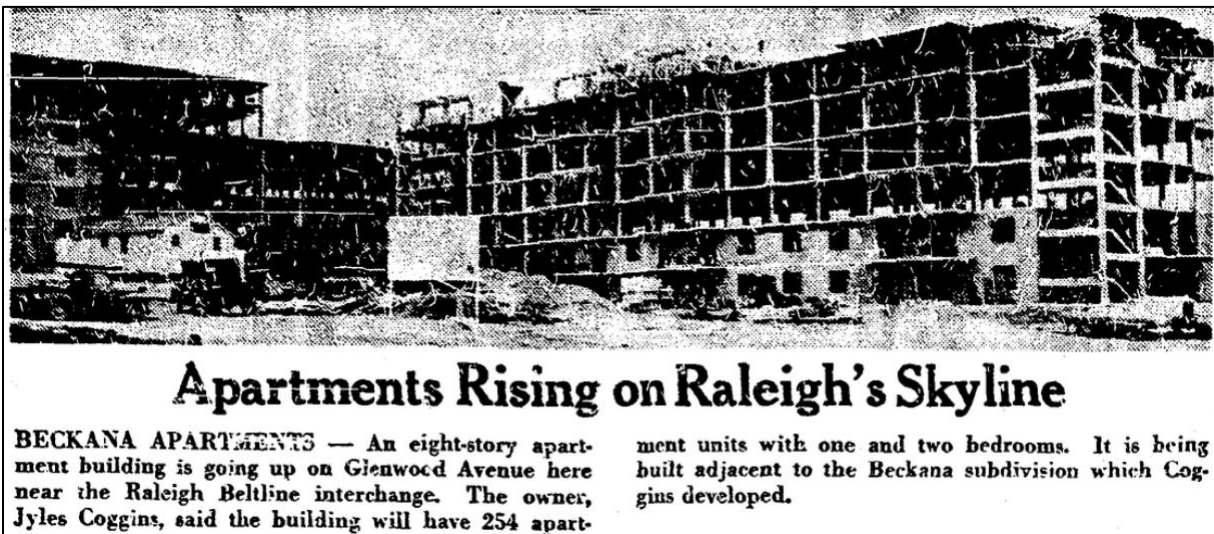
Figure 139: Construction photo of the Beckana Apartments, 1965 ( News and Observer , February 23, 1965).
