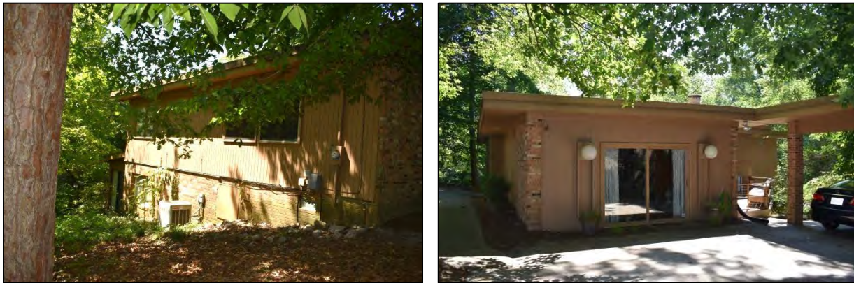
Figure 78: Left, view of eastern elevation; right, view of western elevation
