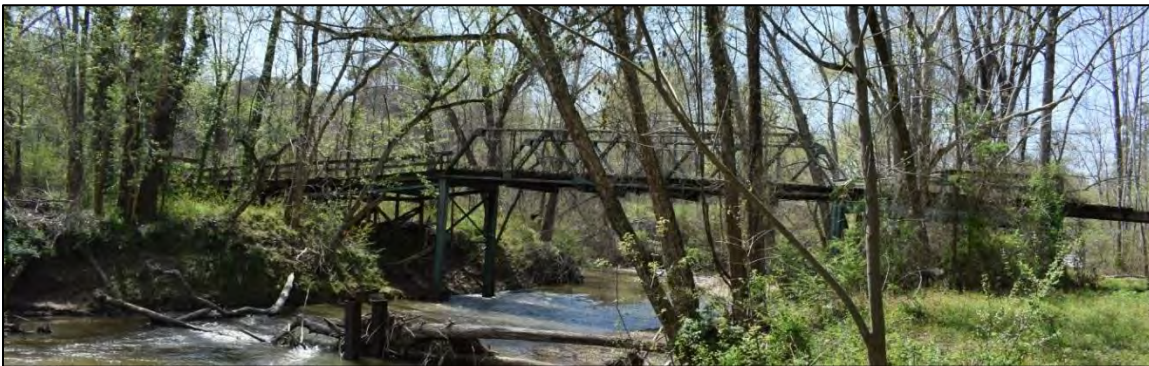
Figure 88: Looking southwest at truss and approach spans
