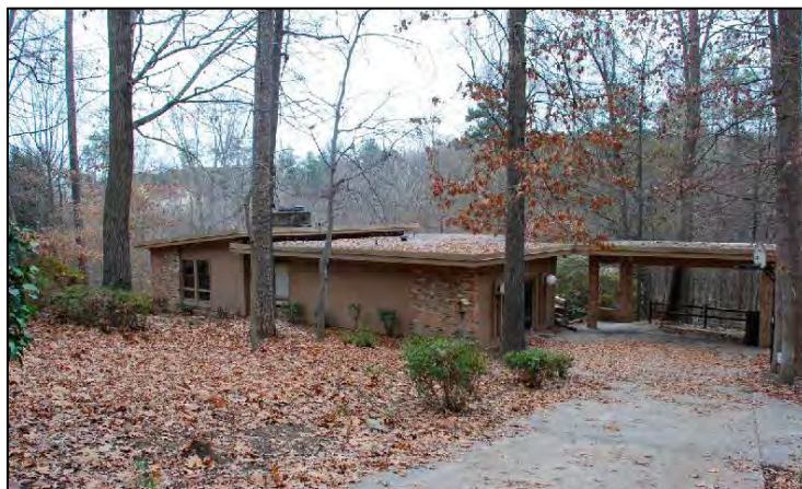
Figure 79. Undated winter view of north front and west side elevations of Harrod House (source: http://www.ncmodernist.org/raleigh.htm )
