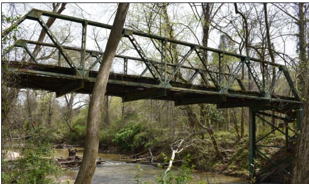
Figure 89: Looking southeast at truss
