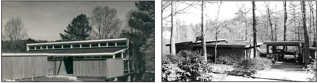
Figure 7: Left, Leroy Martin House (source: http://www.ncmodernist.org/shawcroft.htm ); right, Harrod House, photographed by Sara Lachenman in 2006 (WA4643 survey file)
