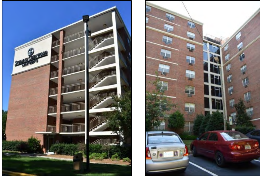
Figure 132: Left, view of eastern (primary) elevation of southern building; right, view of hyphen connecting northern and southern buildings
