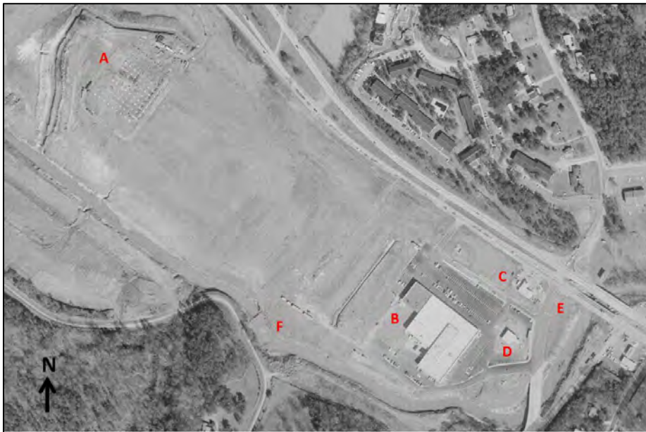
Figure 123: February 1971 USDA aerial capturing mall near onset of construction
