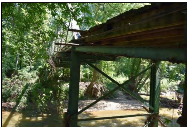
Figure 92: At left, looking northeast at approach span substructure and truss from south bank of Crabtree Creek; at right, looking northwest at steel floor beams, wood floor beams, and V-laced members of truss
