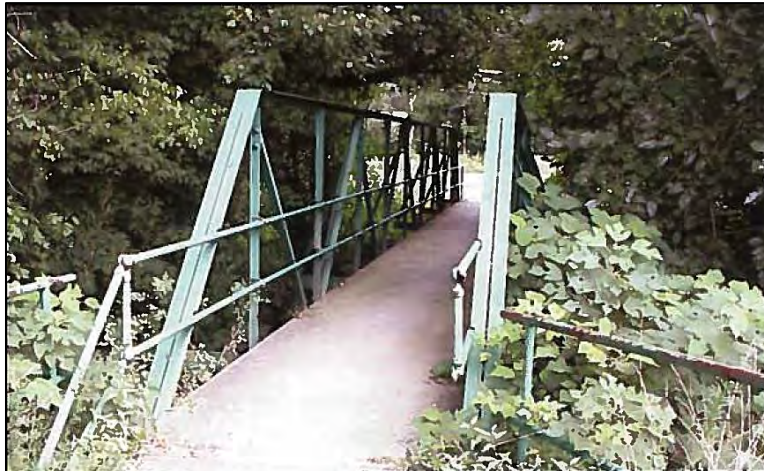
Figure 101: Liberia Street Footbridge (Forsyth County & Winston Salem 2008:113)
