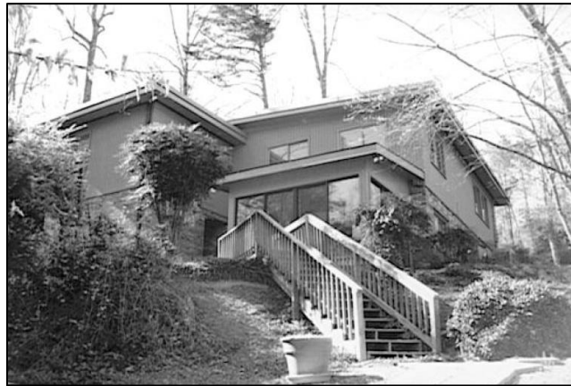
Figure 81: South rear and east side elevations of house in late winter, 2006 (Harrod House File, NC SHPO; photographer: Sara Lachenman)
