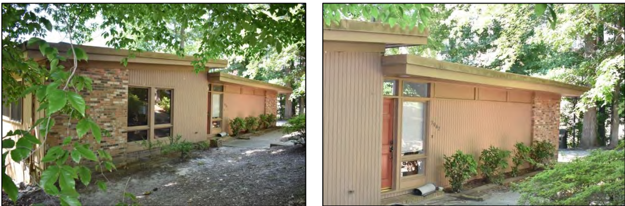
Figure 77: Left, north front elevation with eastern block at left; right, western block with entry and painted clerestory windows
