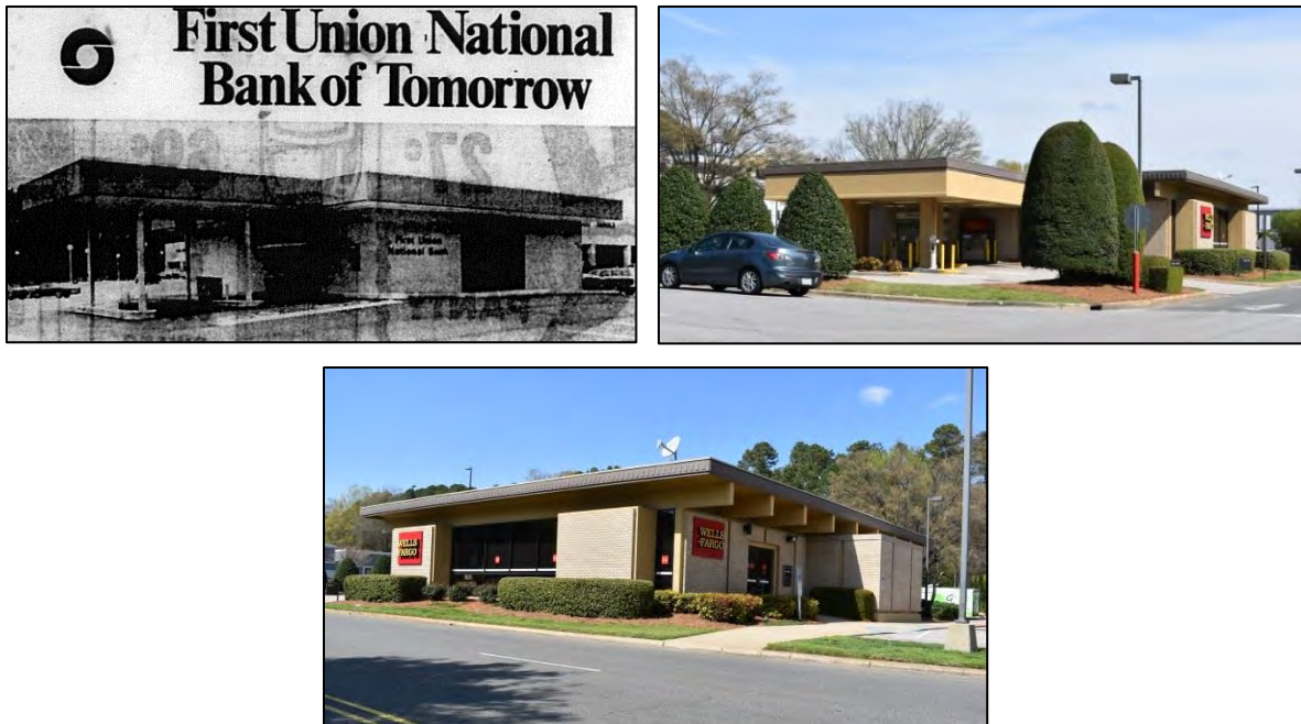
Figure 115: Looking west at First Union, now Wells Fargo Bank, at the mall's opening ( News and Observer , August 2, 1972), upper left, and at present, upper right; looking north at bottom
