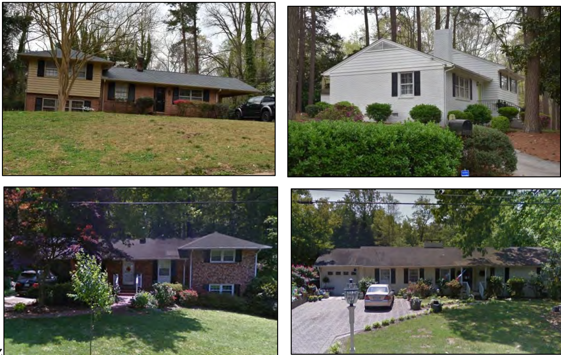
Figure 28: 2007 Varnell Avenue [1959] at top left and 1811 Varnell [1958] at top right; 1909 Manuel Street [1960] at bottom left and 1813 Manuel [1960] at bottom right
