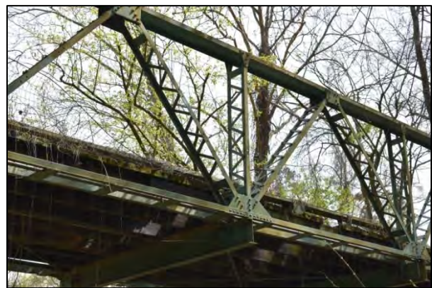
Figure 92: At left, looking northeast at approach span substructure and truss from south bank of Crabtree Creek; at right, looking northwest at steel floor beams, wood floor beams, and V-laced members of truss
